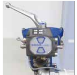
DOUBLE FILTER AND DIFFERENTIAL PRESSURE CONTACT DISPLAY for cooling water
