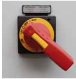
MAIN SWITCH according to VDE installed in attached cabinet.
